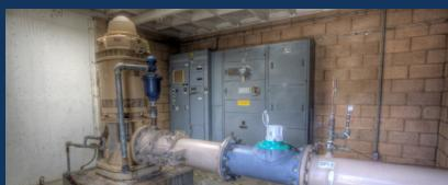
The District is rehabilitating Well No. 2 to improve its efficiency, overall performance and ensure a sustainable and safe water supply. To do this, the project begins with inspections and clean-up of any sediments that have accumulated over time. The pump and motor system are evaluated for replacement or repairs along with piping and electrical system upgrades.
